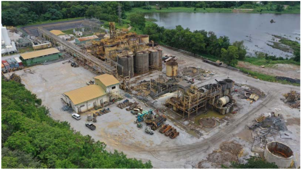
Process plant dismantling
