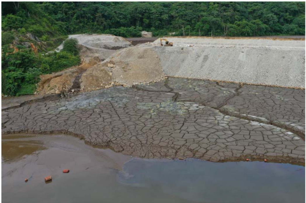
Tailings stabilisation by lowering storage levels behind the retaining embankments
